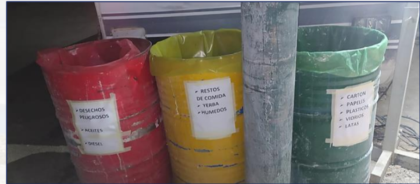
Onsite Waste Separation
