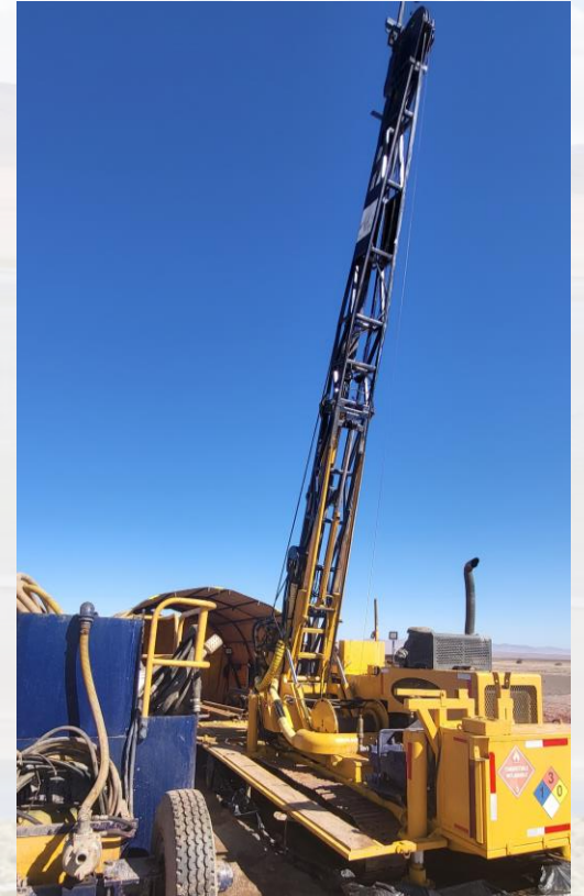
Drill Rig on POZO LL-01, Molle Verde
