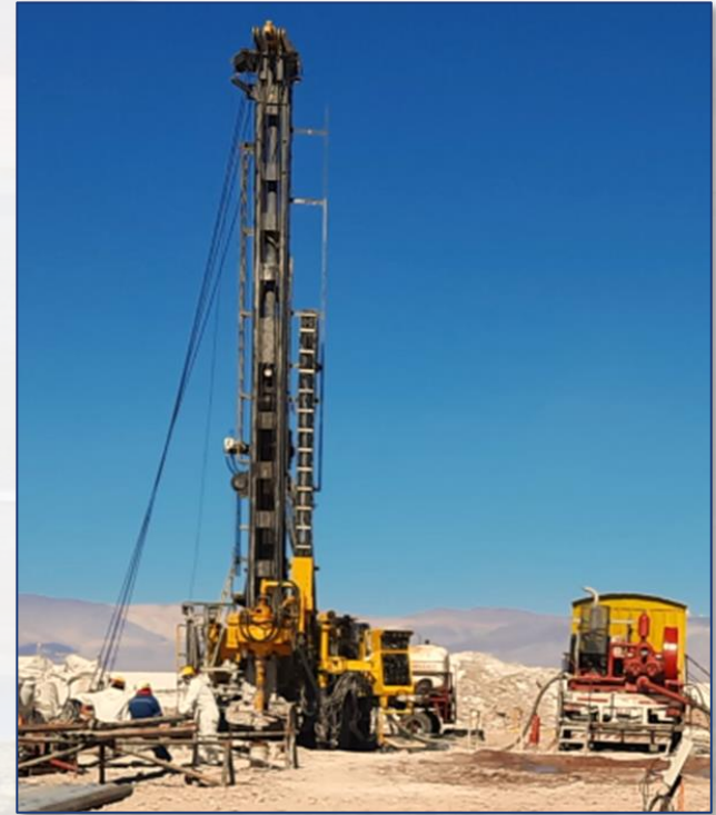
Drill Rig on the Salar Arizaro
